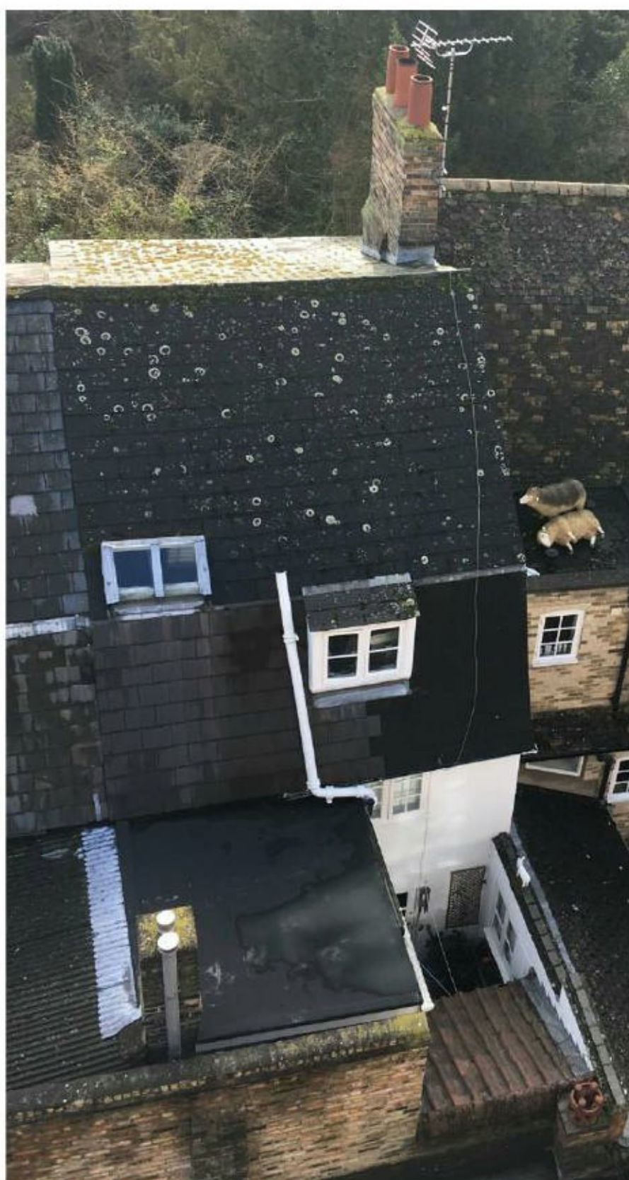
Figure 8: 9 Little St Mary's Lane (centre of photo)
