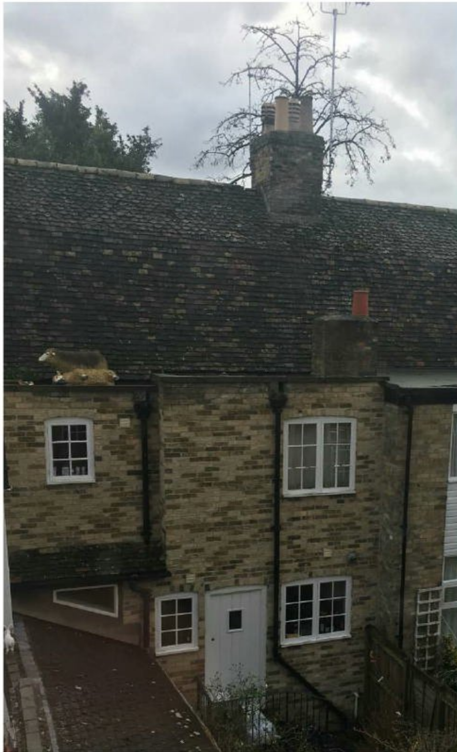
Figure 9: 10 Little St Mary's Lane (centre of photo)
