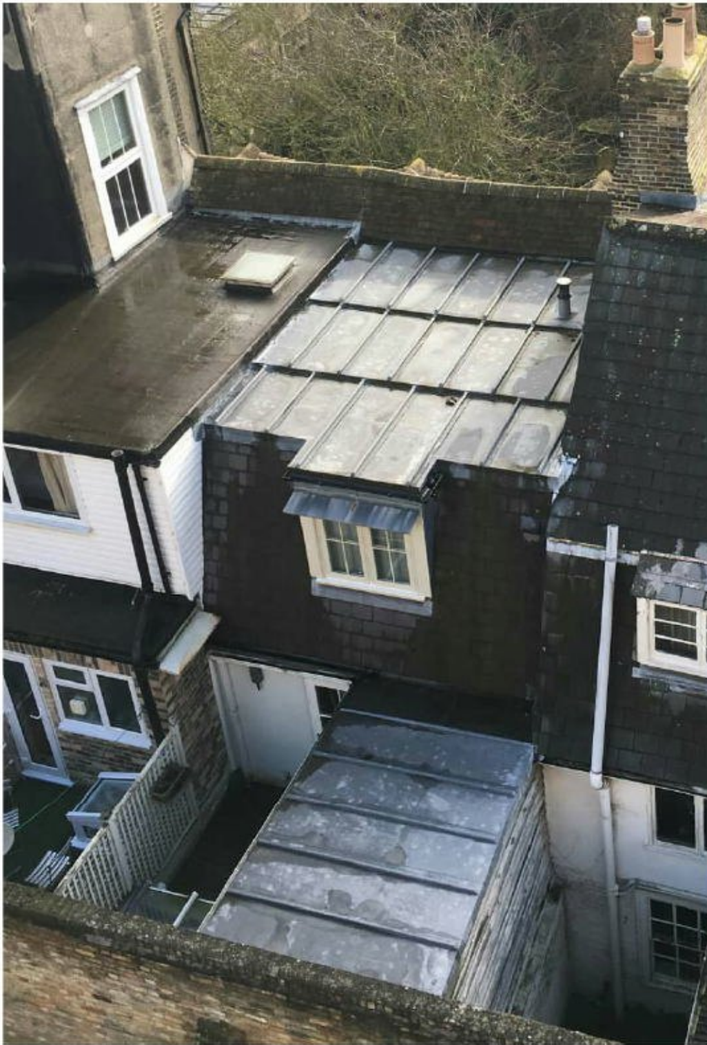
Figure 6: 7 Little St Mary's Lane (centre of photo)
