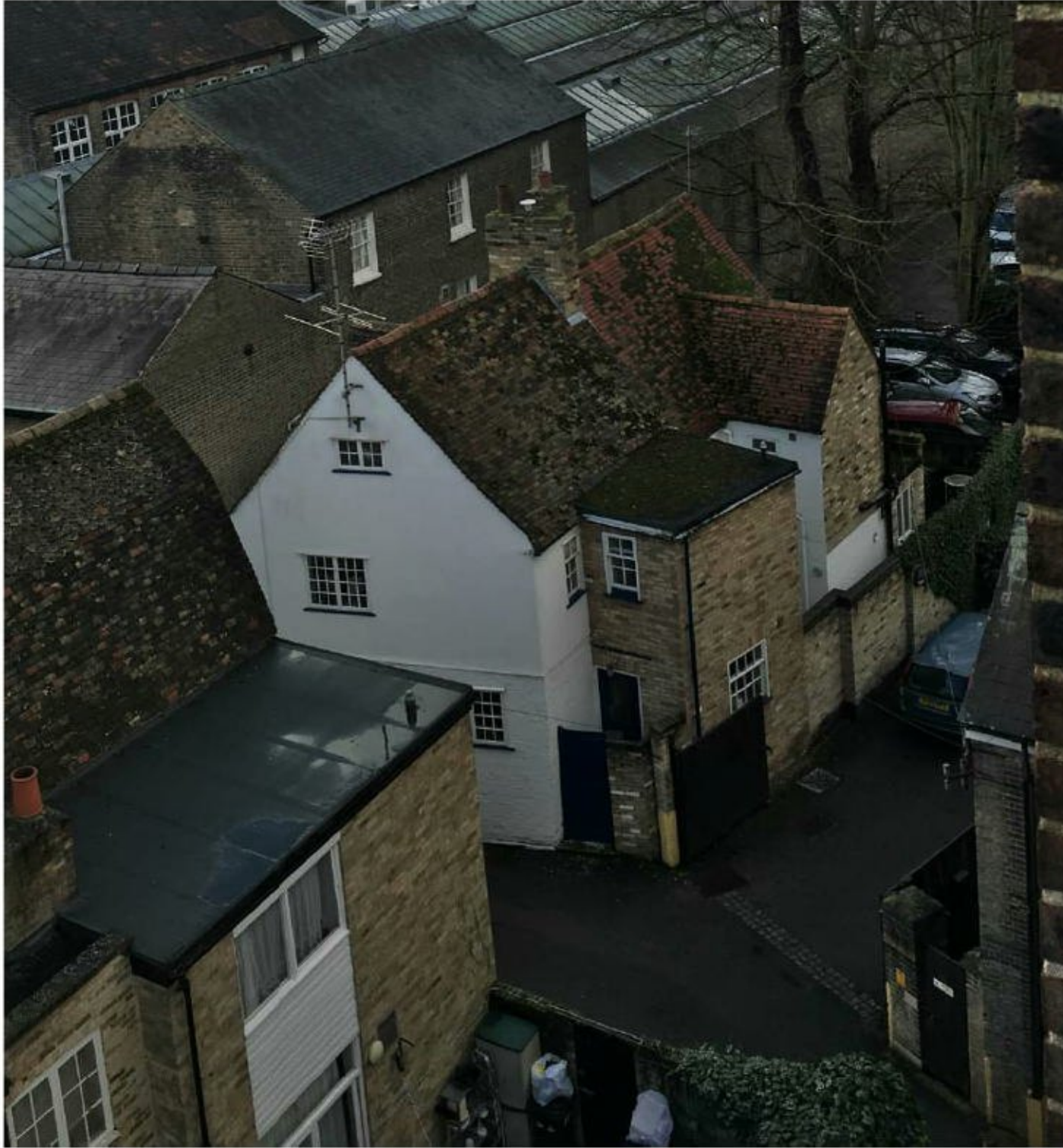
Figure 10: 11 Little St Mary's Lane (left of photo)
