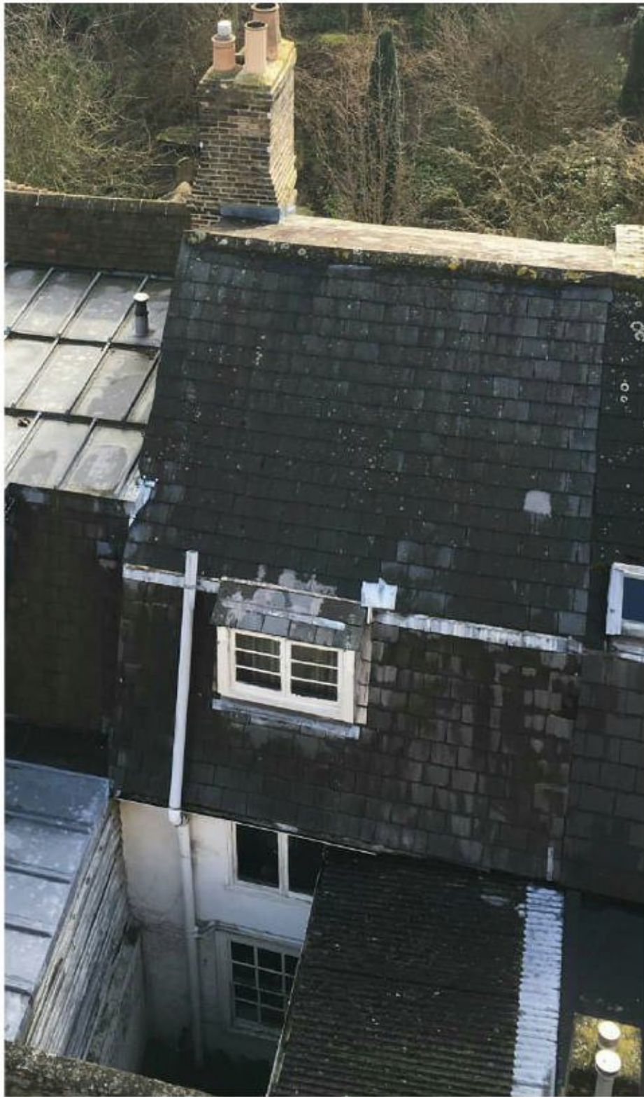
Figure 7: 8 Little St Mary's Lane (centre of photo)
