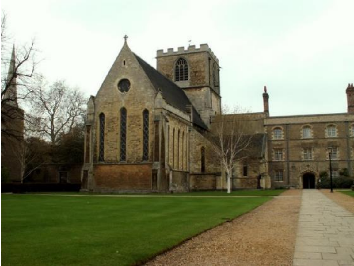
Figure 13: View of the Chapel
