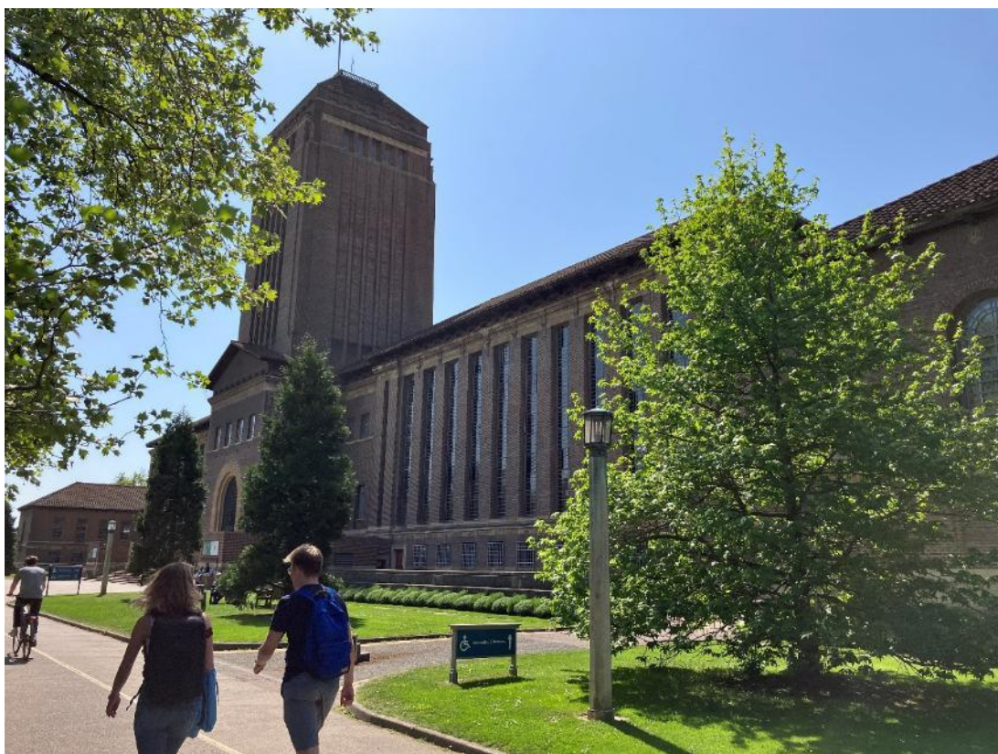
Figure 36 - View of Cambridge Library
